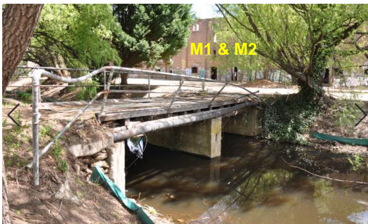
Figure 6 - Bridge to be used for sewer rising main and watermain crossing of Nattai River
