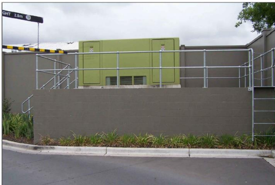
Figure 16 - Example of Pad Mount Substation raised clear of the 1:100 year flood level
